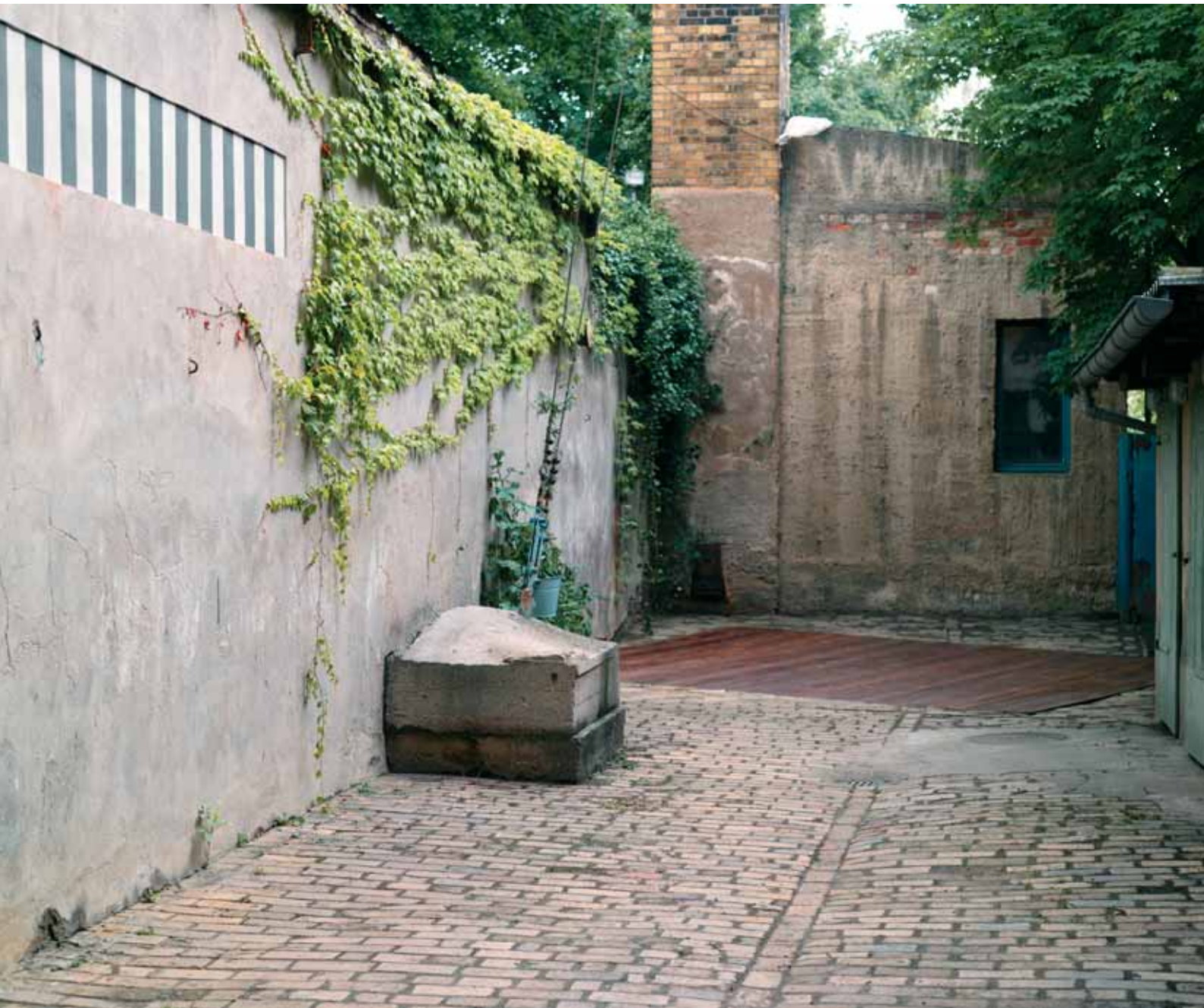
Karl-Heine-Str. 43, inner courtyard, 2008
